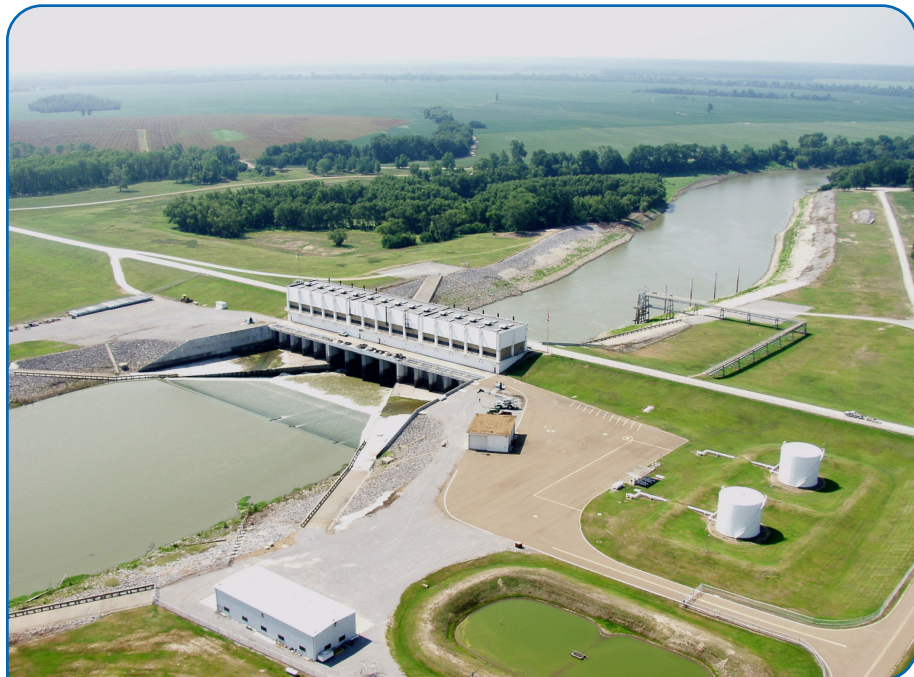
Memphis District’s W.G. Huxtable Pumping Station.
