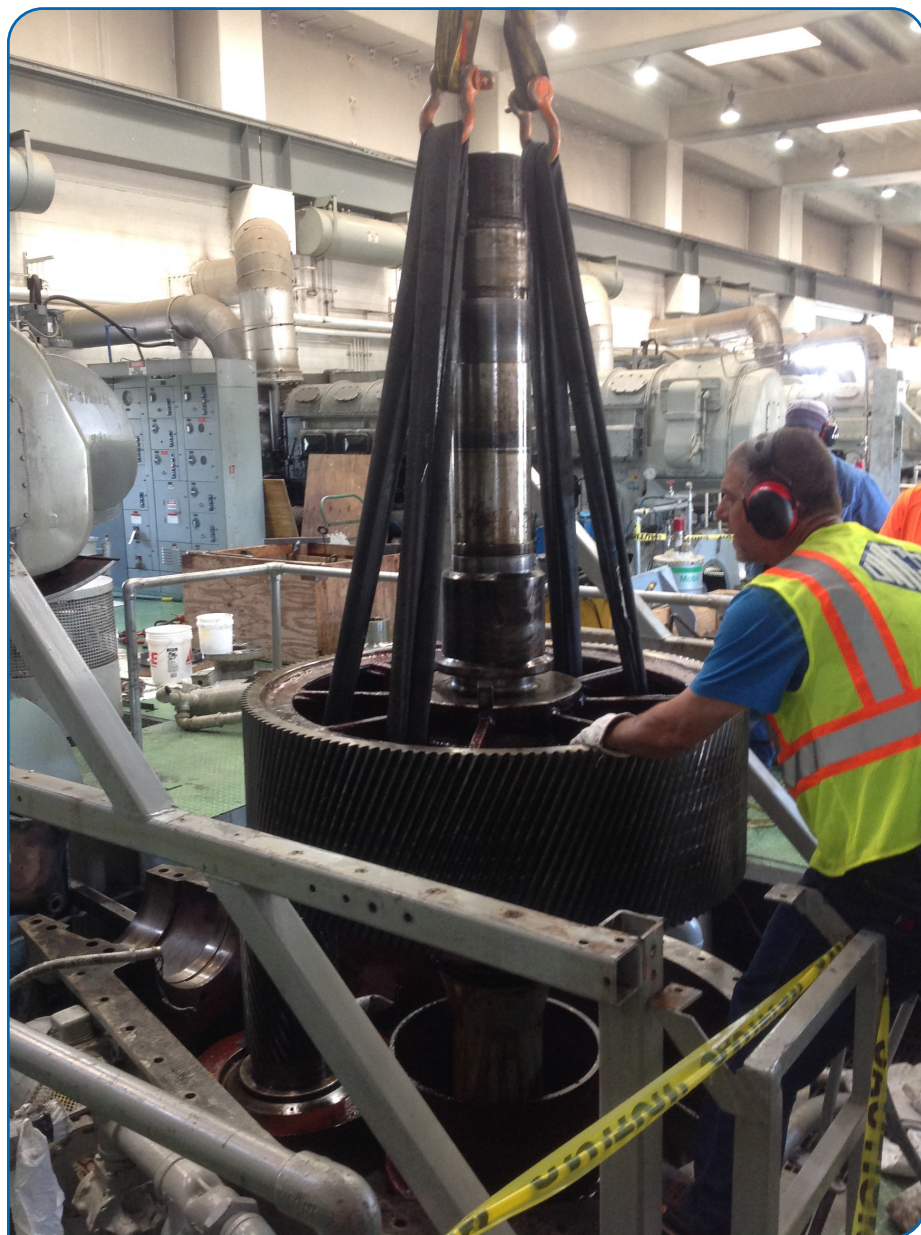
Disassembly and removal of one of the gearboxes.
