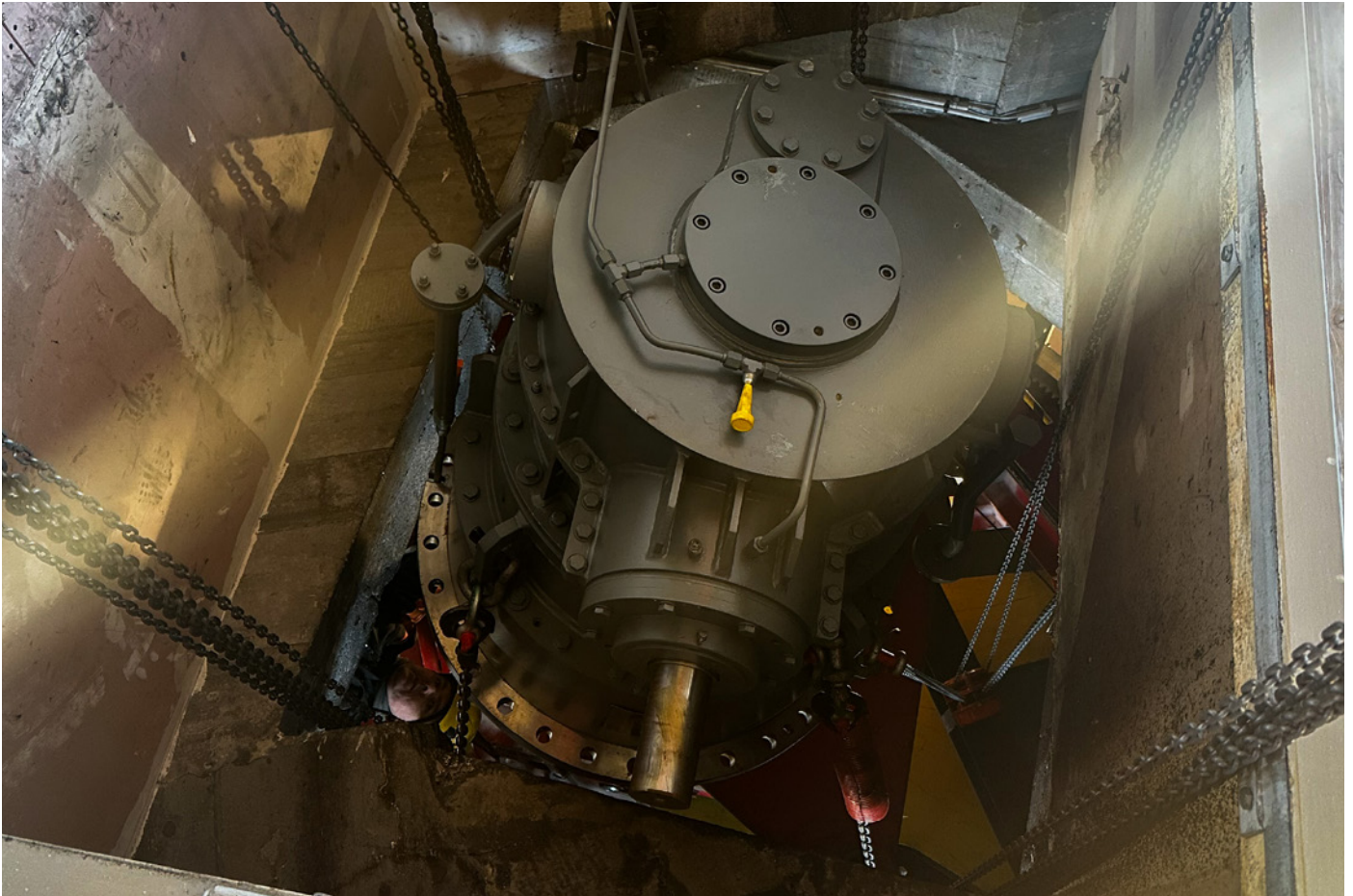
The new replacement gearbox came with newer technology and better materials than previous versions.
