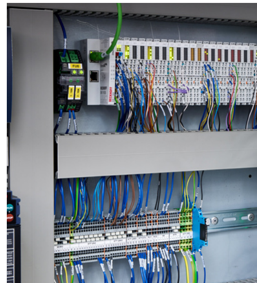
The C6920 control cabinet Industrial PC (right), which runs the TwinCAT CNC for up to twelve servo axes and spindles, and the associated EtherCAT Terminal system (left).
