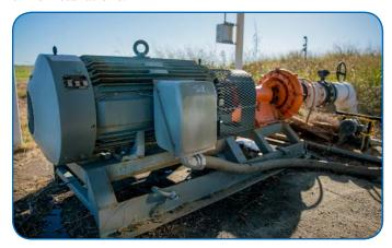
Featuring a totally-enclosed fan-cooled design in a cast iron frame, this proven design is suitable for indoor or outdoor installation in some of the most demanding environments and applications. Rated as a 100 hp, 460 v, 1,800 rpm electric motor, this innovative design delivers 95.5% efficiency at rated load with a near-unity power factor. The NEMA 449T frame motor weighs about 2,700 pounds and draws just 170 amps at full load.
