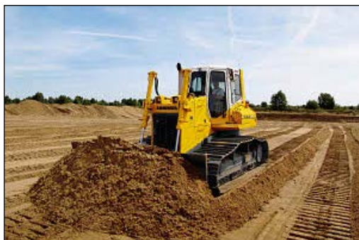
Figure 9 Excavator and scraper (Source: Liebherr).
