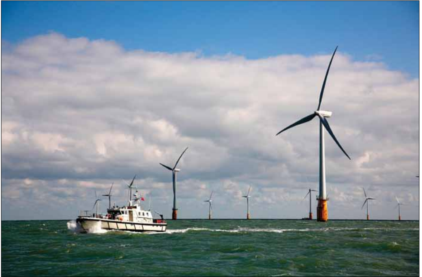
The Thanet Offshore Wind Farm is currently the largest offshore farm operating in the world (courtesy of Vattenfall).
