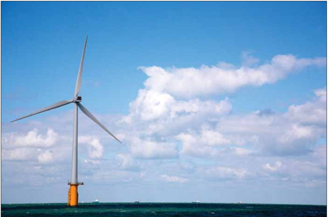
The Thanet project was completed in September 2010 and will boost offshore capacity by 30 percent (courtesy of Vattenfall).
