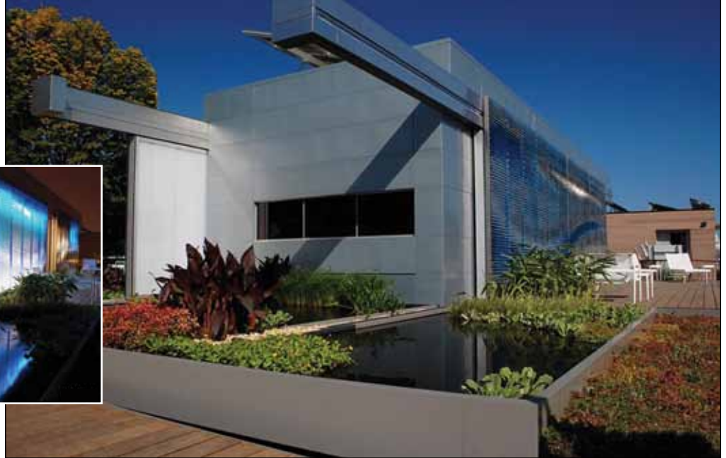
Lumenhaus is Virginia Tech University's 800-square-foot, energy-optimized "smart" home that has the ability to maintain optimal energy performance at all times. It leverages an active system of motion controls from Thomson and Kollmorgen (courtesy M. Cincala).
