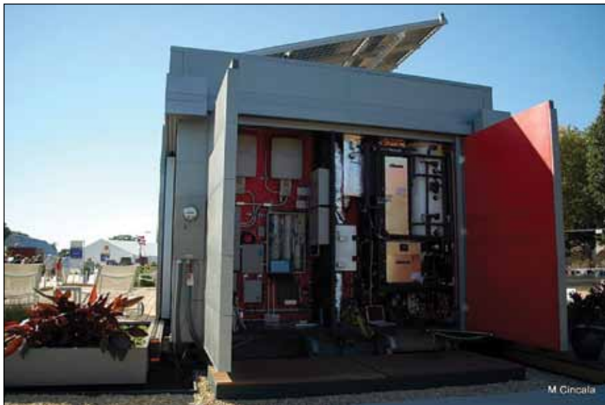
All of Lumenhaus’s components and systems are designed and built to work together to maximize user comfort with environmental protection. At its heart is an integrated, environmental control system (courtesy M. Cincala).
