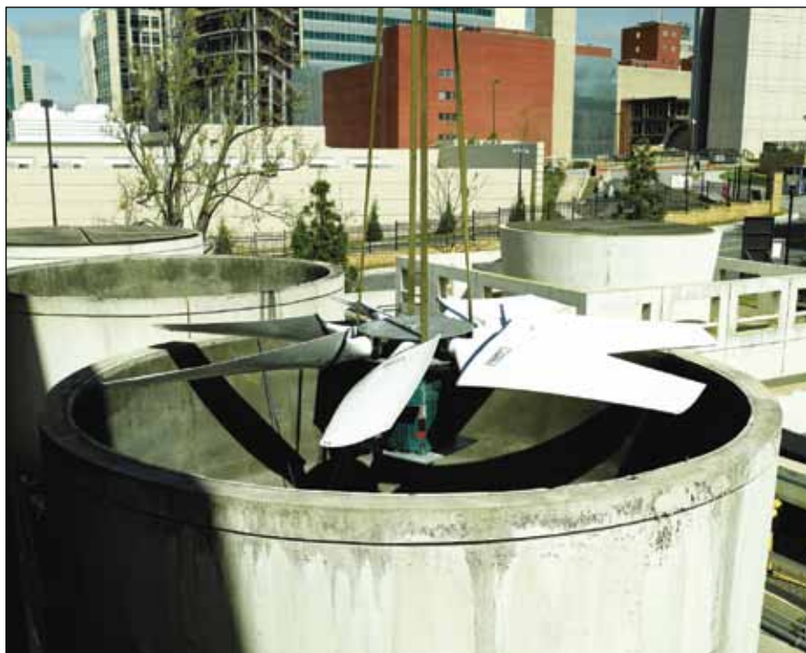
The Baldor Reliance RPM AC Cooling Tower Direct Drive Motor is designed exclusively for the cooling tower industry. This motor combines the technologies of the power-dense, laminated frame RPM AC motor with high performance, permanent magnet salient pole rotor designs (photos courtesy of Baldor).
