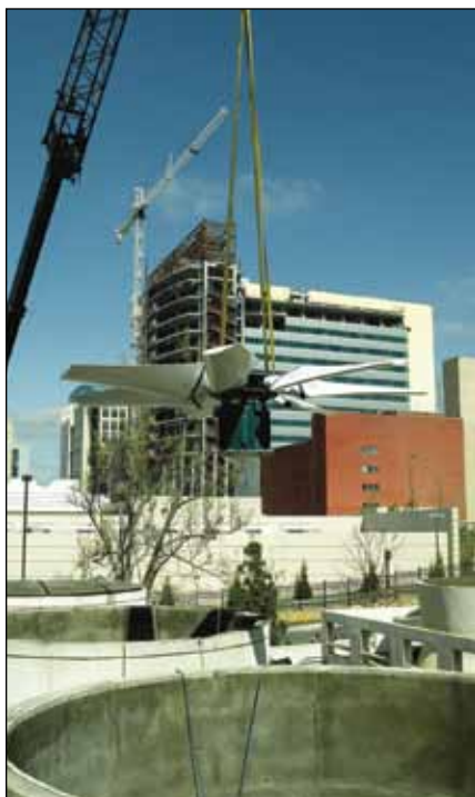
The Baldor Reliance RPM AC Cooling Tower Direct Drive Motor is designed exclusively for the cooling tower industry. This motor combines the technologies of the power-dense, laminated frame RPM AC motor with high performance, permanent magnet salient pole rotor designs (photos courtesy of Baldor).
